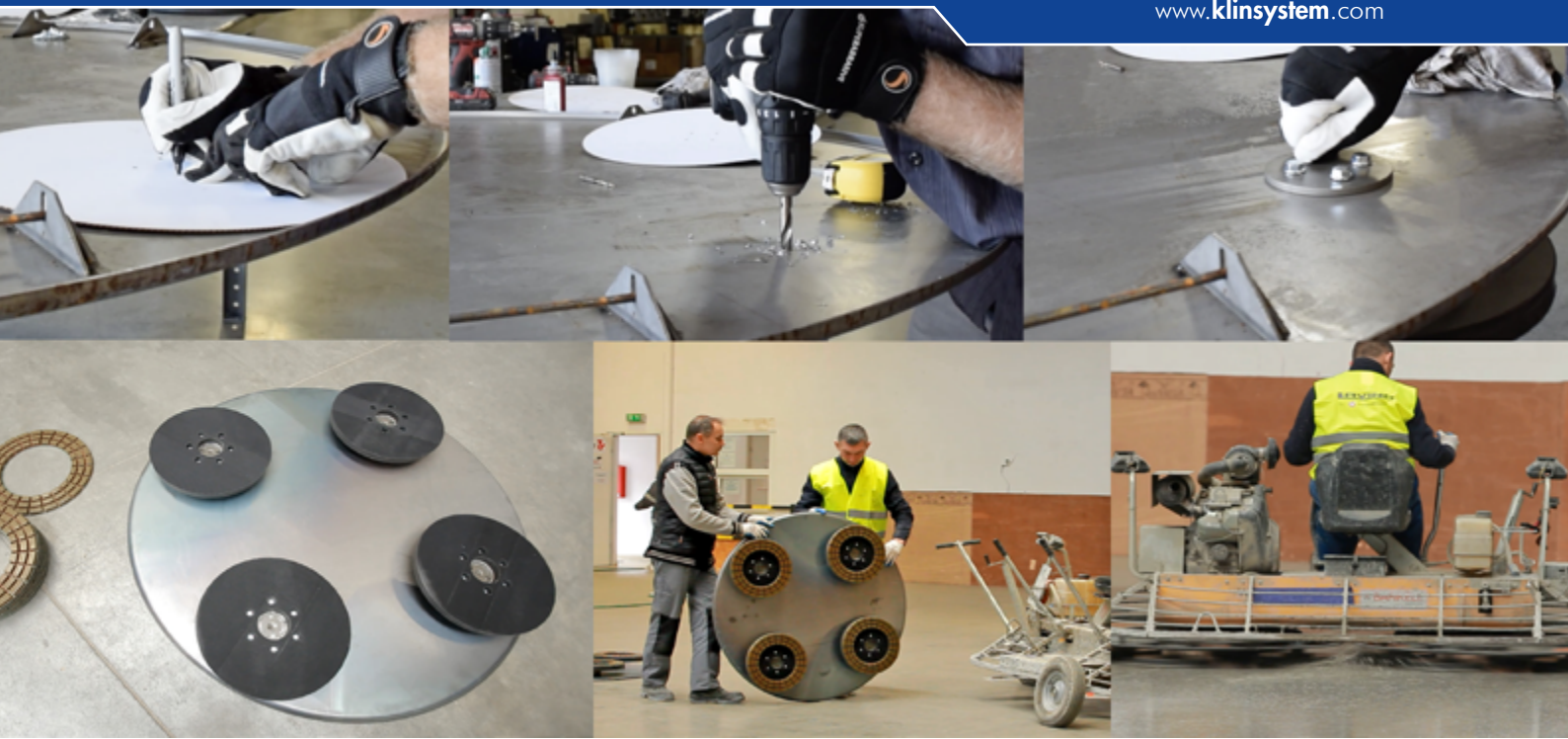
Installation of velcro pad holders on the floating pans
